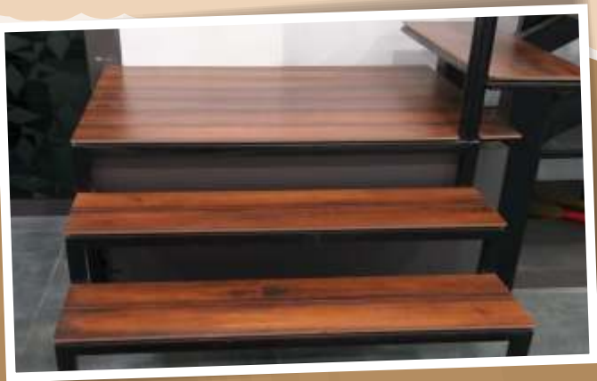
Flooring used in stair case
